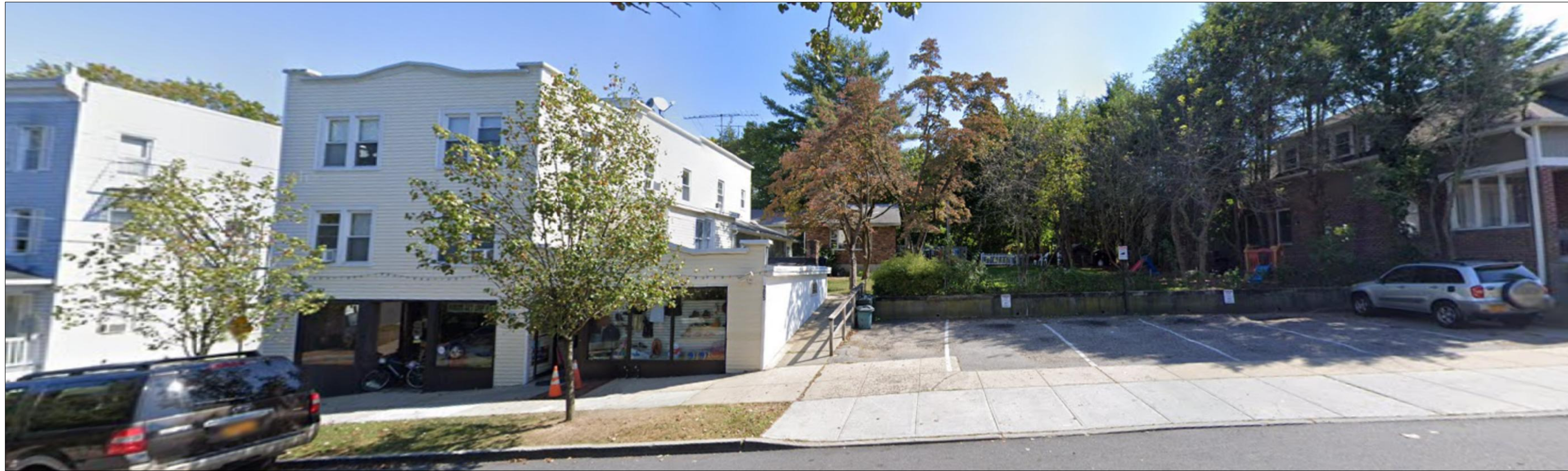
EXISTING STREETScape ALONG LEXINGTON AVENUE
