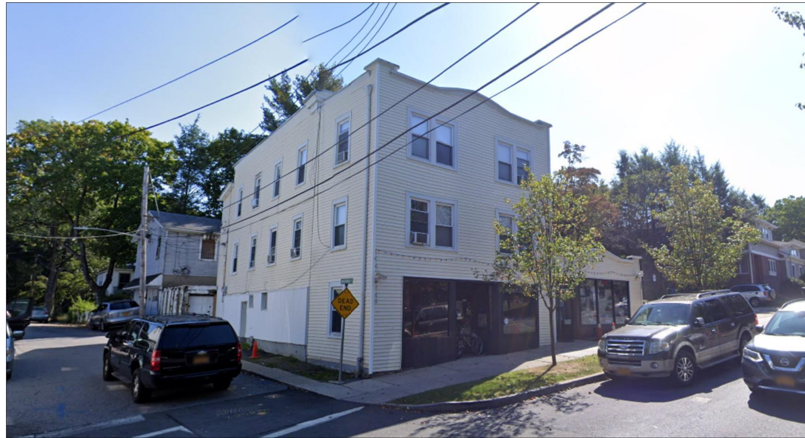
EXISTING STREETScape ALONG MAPLEWOOD AVENUE
