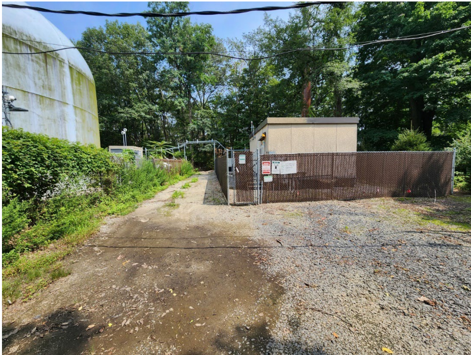
Equipment compound area. Monopole shown behind the tan equipment shed. Village water tank at left.
